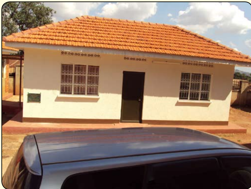
Exterior of Newly renovated laboratory of Nsambya home care
